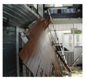
The figure on the left shows a collapsed roof due to inadequate restraints provided by nail fixings. Corrosion of the nails may have contributed as well. (Picture referenced from an article in QBCC)
